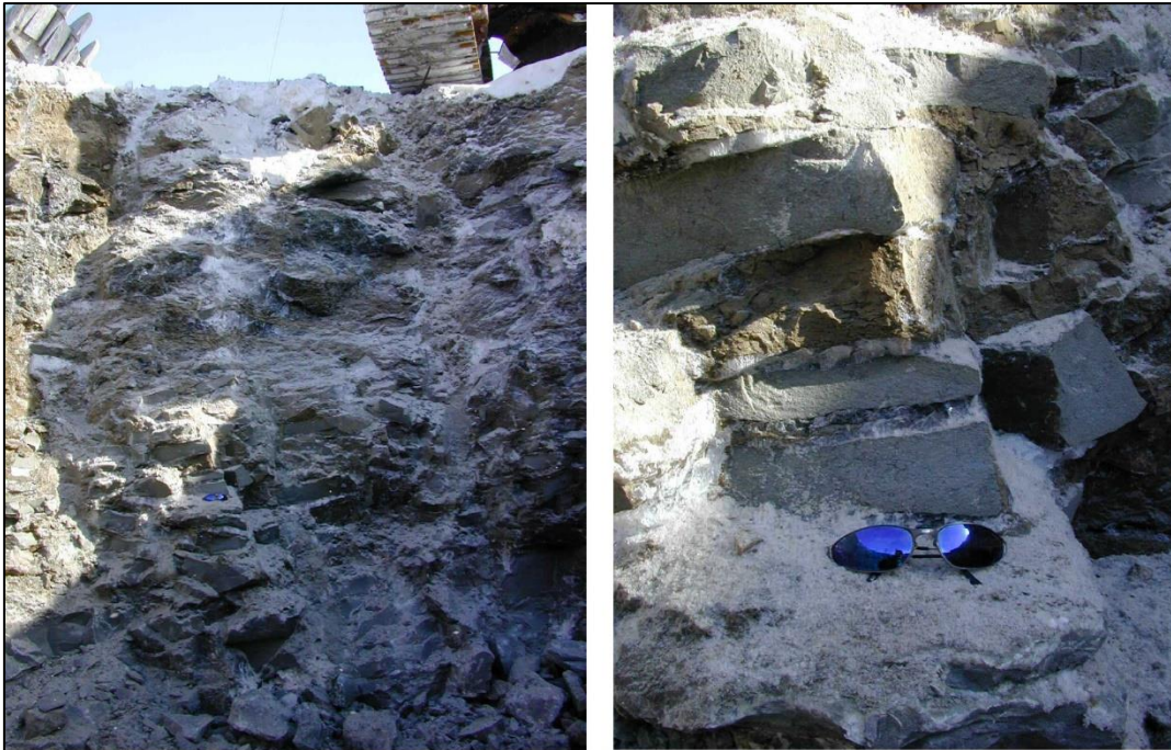
Figure 1 Photo of an excavation for antenna foundations at Platåberget
